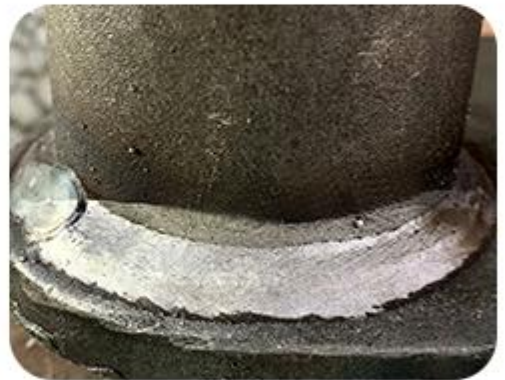
Weld Seam Cleaning
